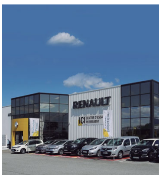
Renault-Nissan dealership with ECO G solution, without causing an increase in energy costs. Romans-sur-Isère, southern France. ECO G
