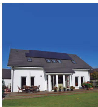
Making the most of the RHI: success with Panasonic heat pump technology. Fife, Scotland. Aquarea
